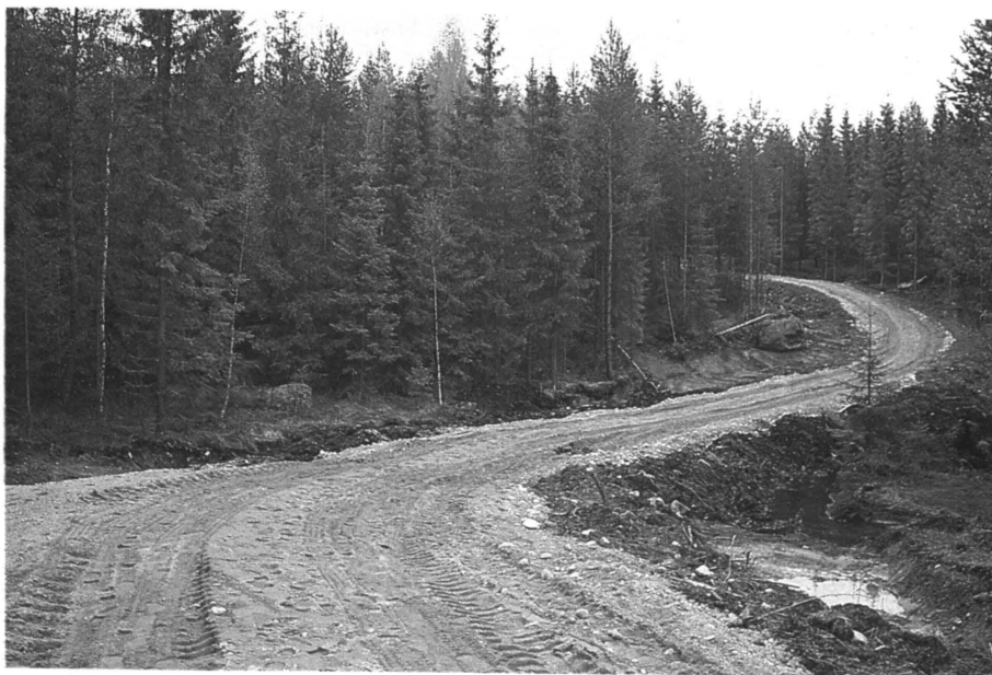
Figure 5. Permanent forest roads serve timber harvesting, silvicultural operations, and multiple use of forests (Photo H. Kalaja).
